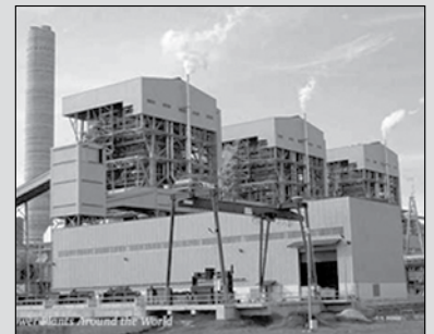
Manjung Power Plant
